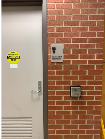
Caption: The Gender Neutral Bathroom in Williams Hall has adequate signage and accessibility.
